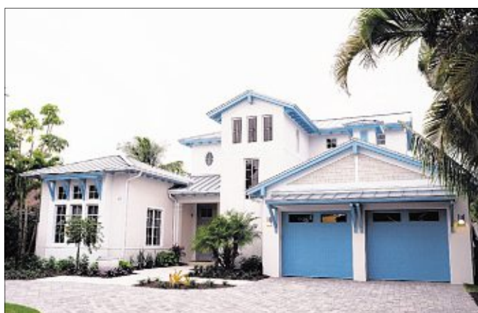
The master bedroom of one of London Bay Homes' model homes, top, and the home's exterior, above. When the recession struck, president and CEO Mark Wilson was forced to cut staff of London Bay Homes from 80 to 20. With the housing market's rebound, he's been able to grow his company once again and now has about 120 employees.
